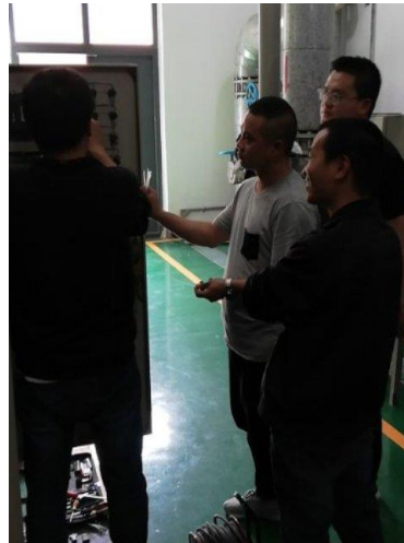
2#交换站更换触摸屏
